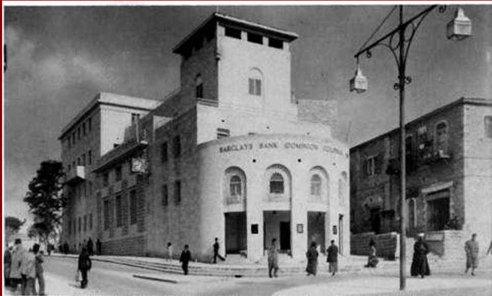
13. The New Municipal Building in Jerusalem, also occupied by Barclay's Bank. The building was usurped in 1948 by the Zionists
